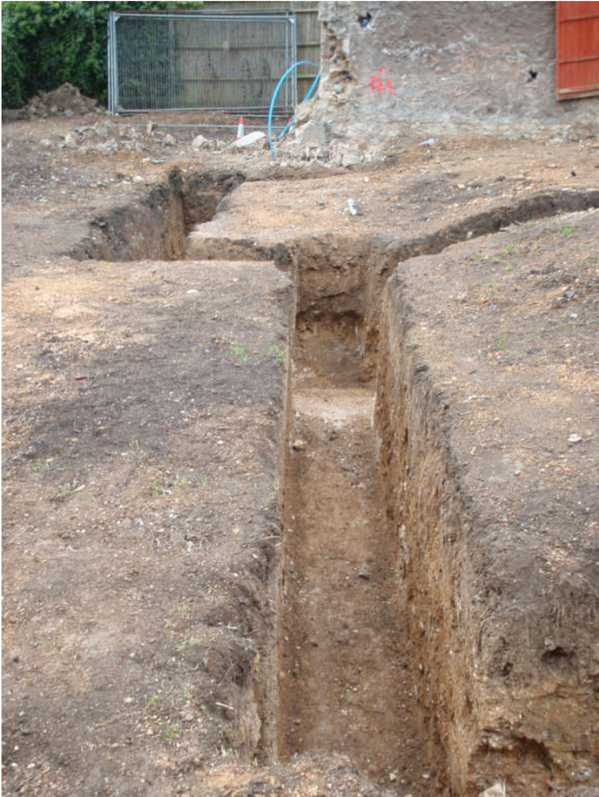
Plate 6. Excavation of foundation trenches (looking west)
