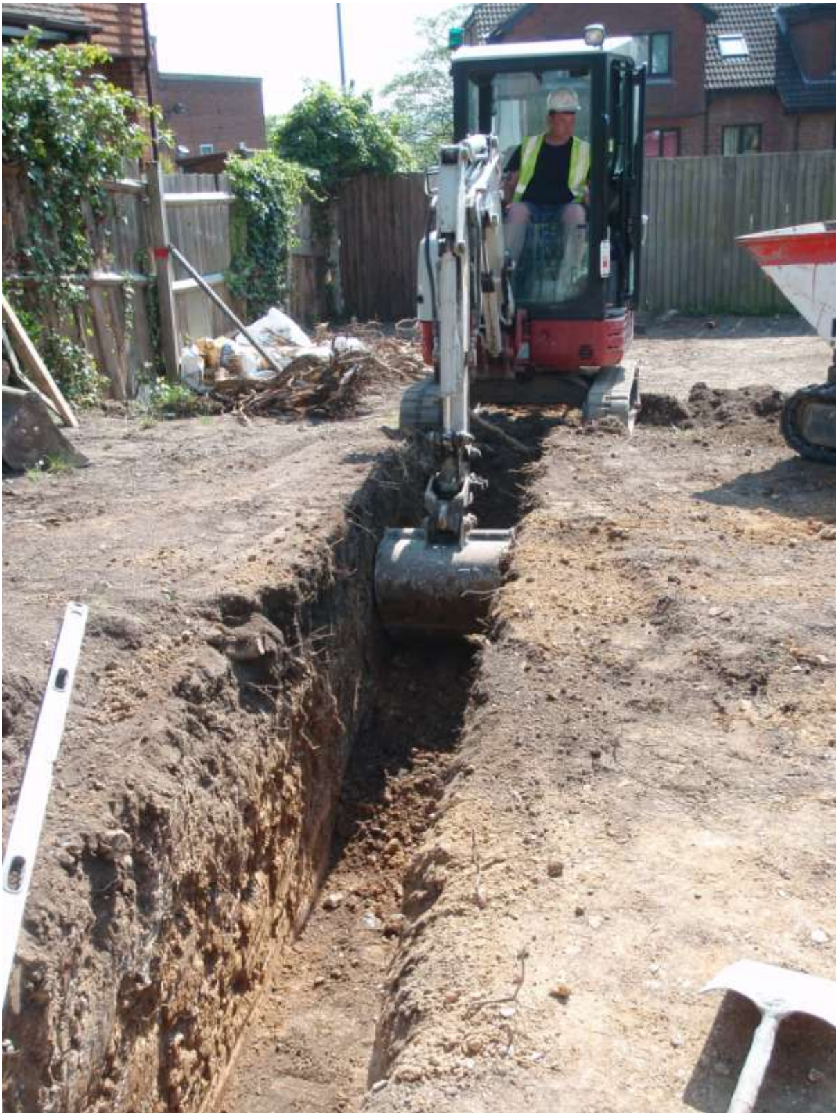
Plate 4. Excavation of foundation trenches (looking south)
