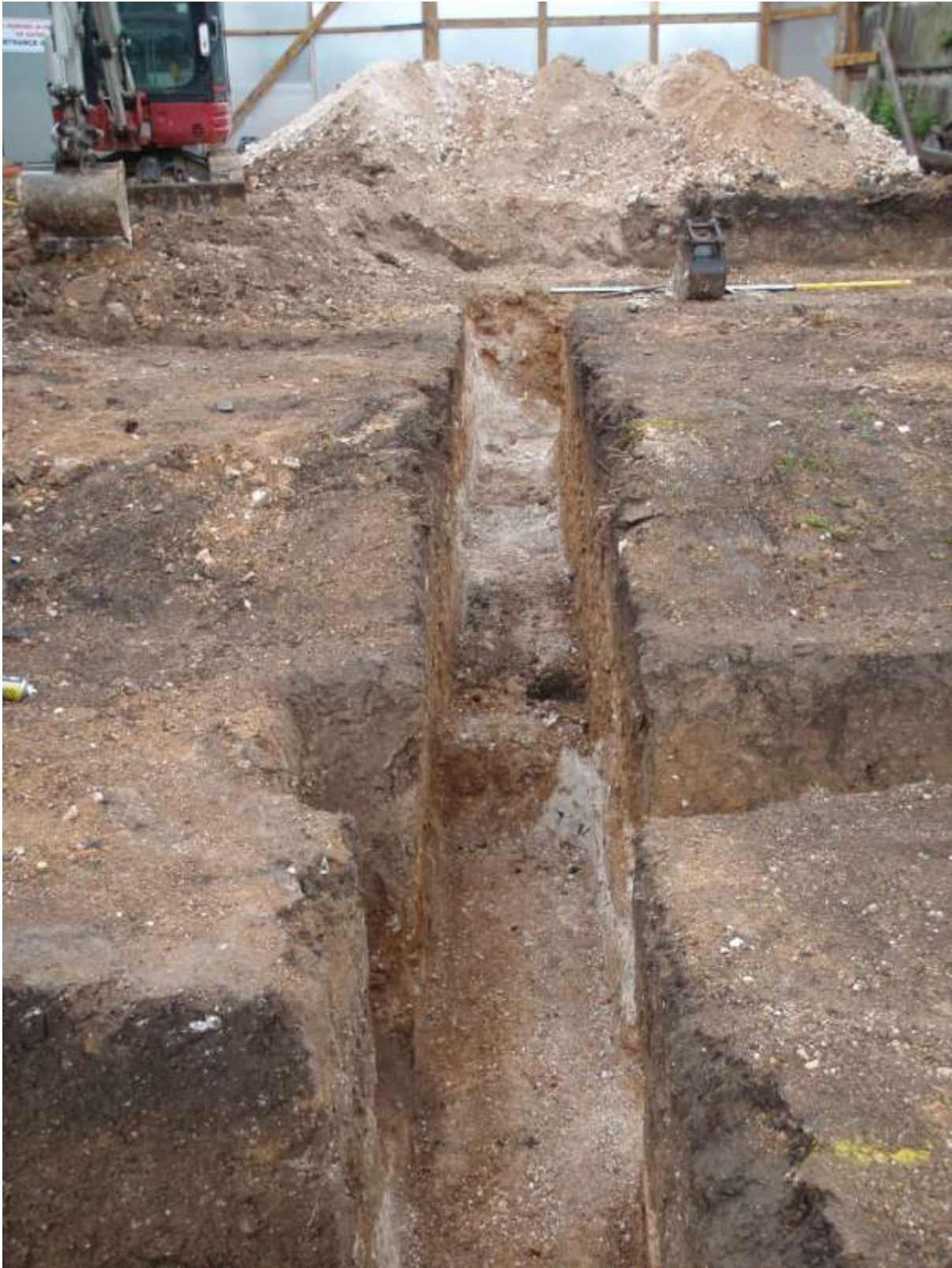
Plate 5. Excavation of foundation trenches (looking north)
