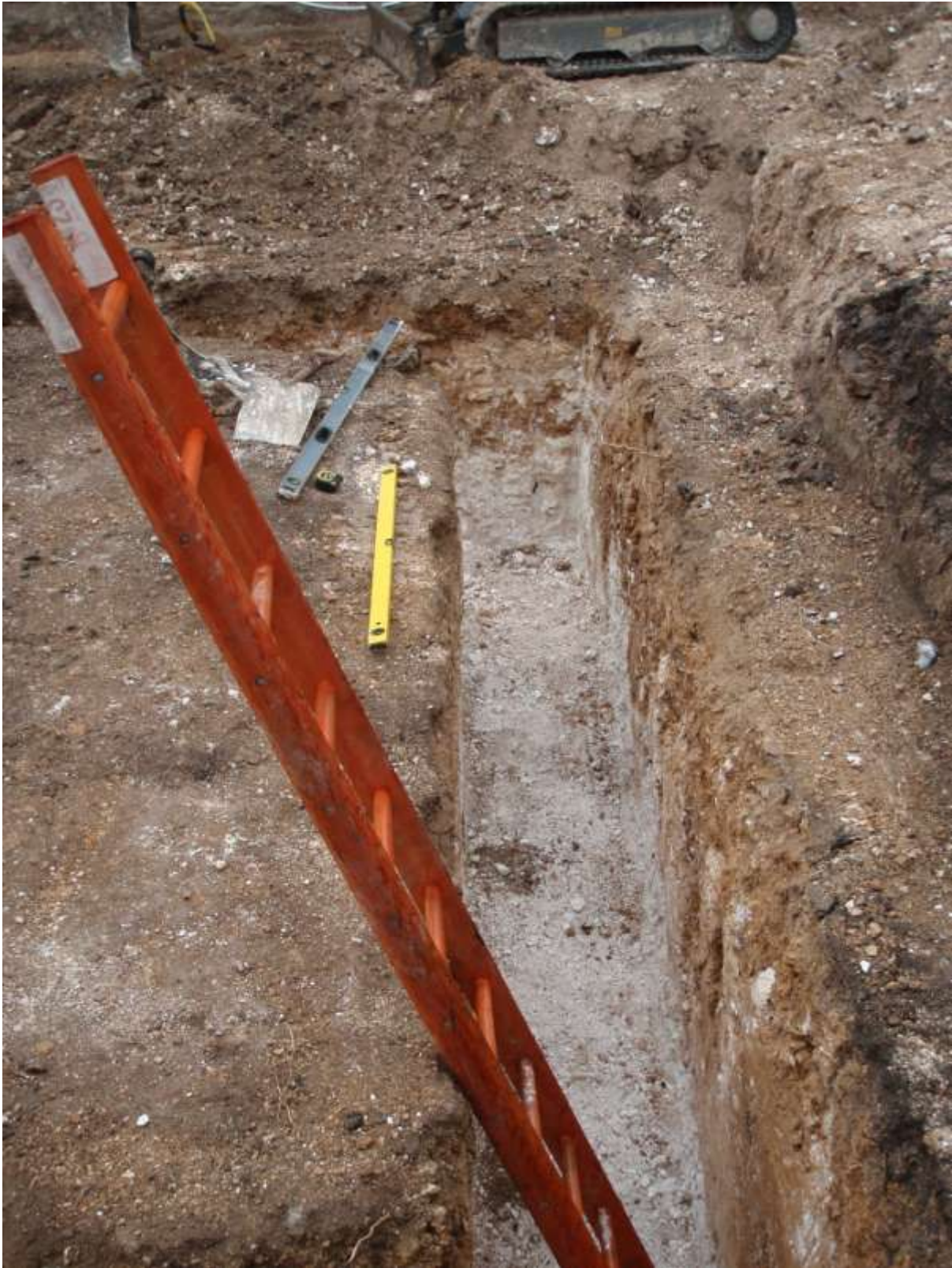
Plate 7. Excavation of foundation trenches (looking north-east)
