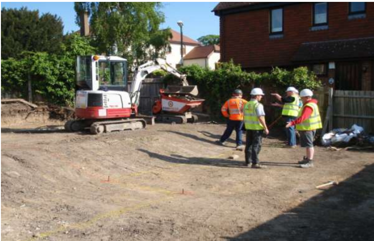
Plate 3. Marking out trench locations (looking north-east)
